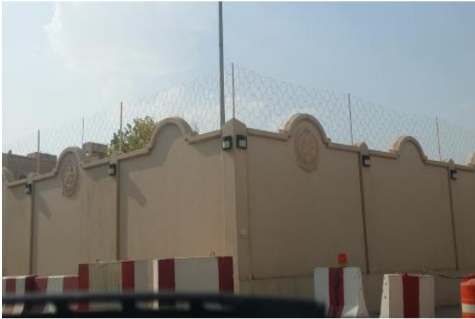
Fiber Optic Mesh Fence on a Military Site Wall
